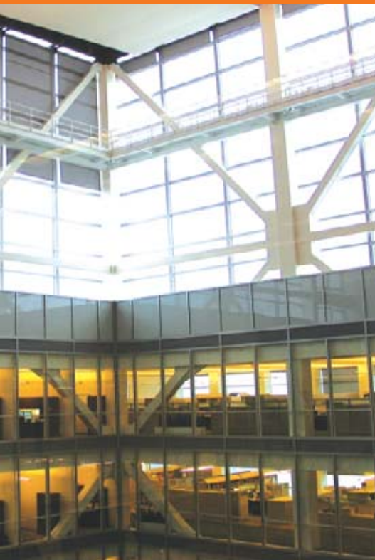
Natural light streams through Union Pacific's 19-story glass atrium. Mechoshade window shades facilitate Union Pacific's "daylighting" strategies
