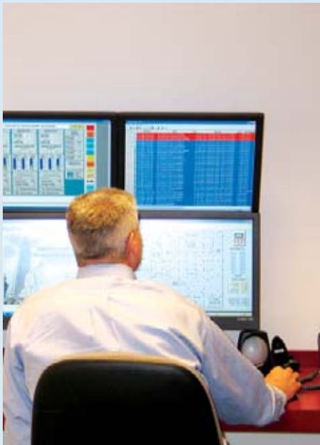
Sam Gibson monitors Union Pacific's building systems from a central CyberStation workstation
